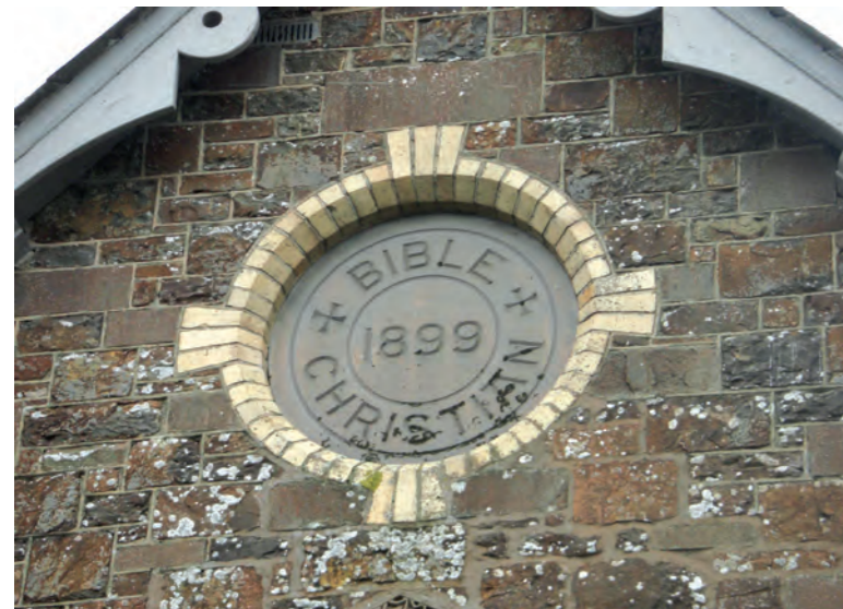
AN INSCRIPTION at the entrance to chapels provides the name and denomination of the chapel as well as the date of the building.
